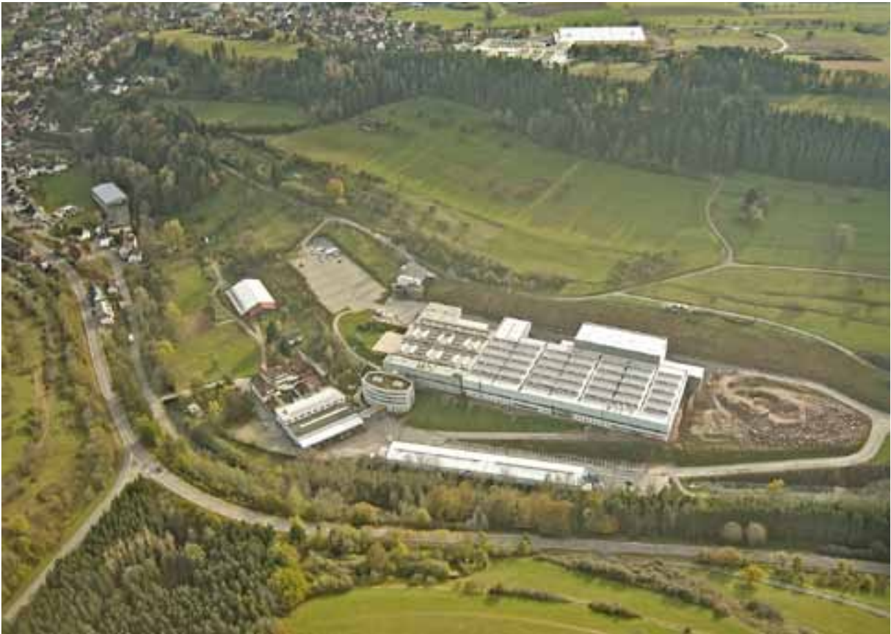
Figure 57 - Areal view of the plant
