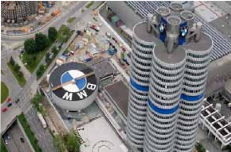
Figure 28 - View of the BMW Headquarters in Leipzig. Supplier of the technology: WDP Windanlage GmbH & Co. KG
