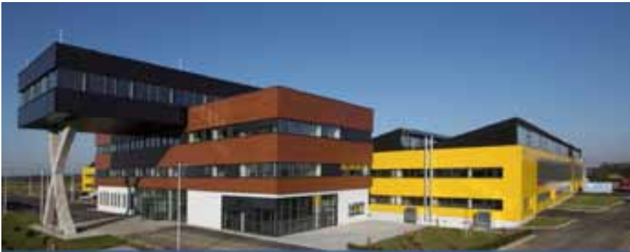
Figure 11 - Office building & production hall of “SUN MASTER”
