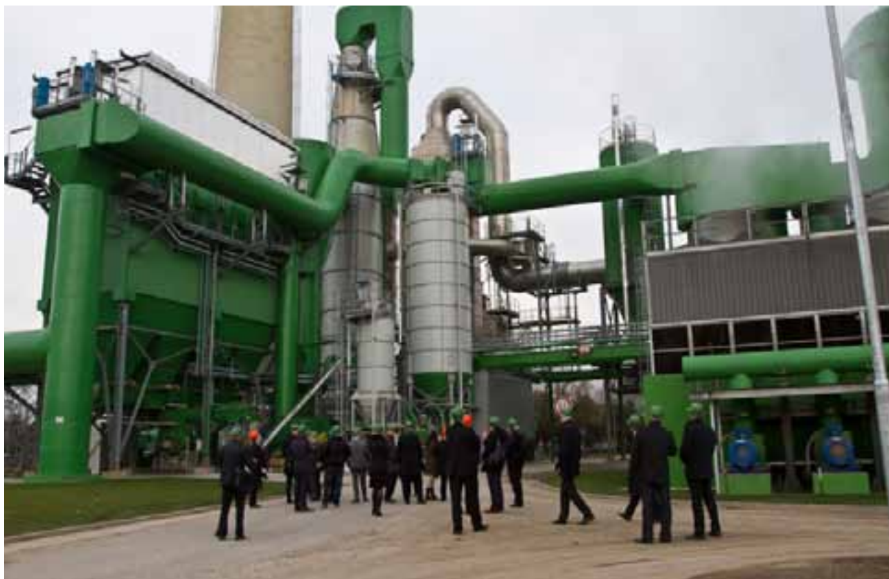
Figure 55 - View of Kosit after reconstruction
