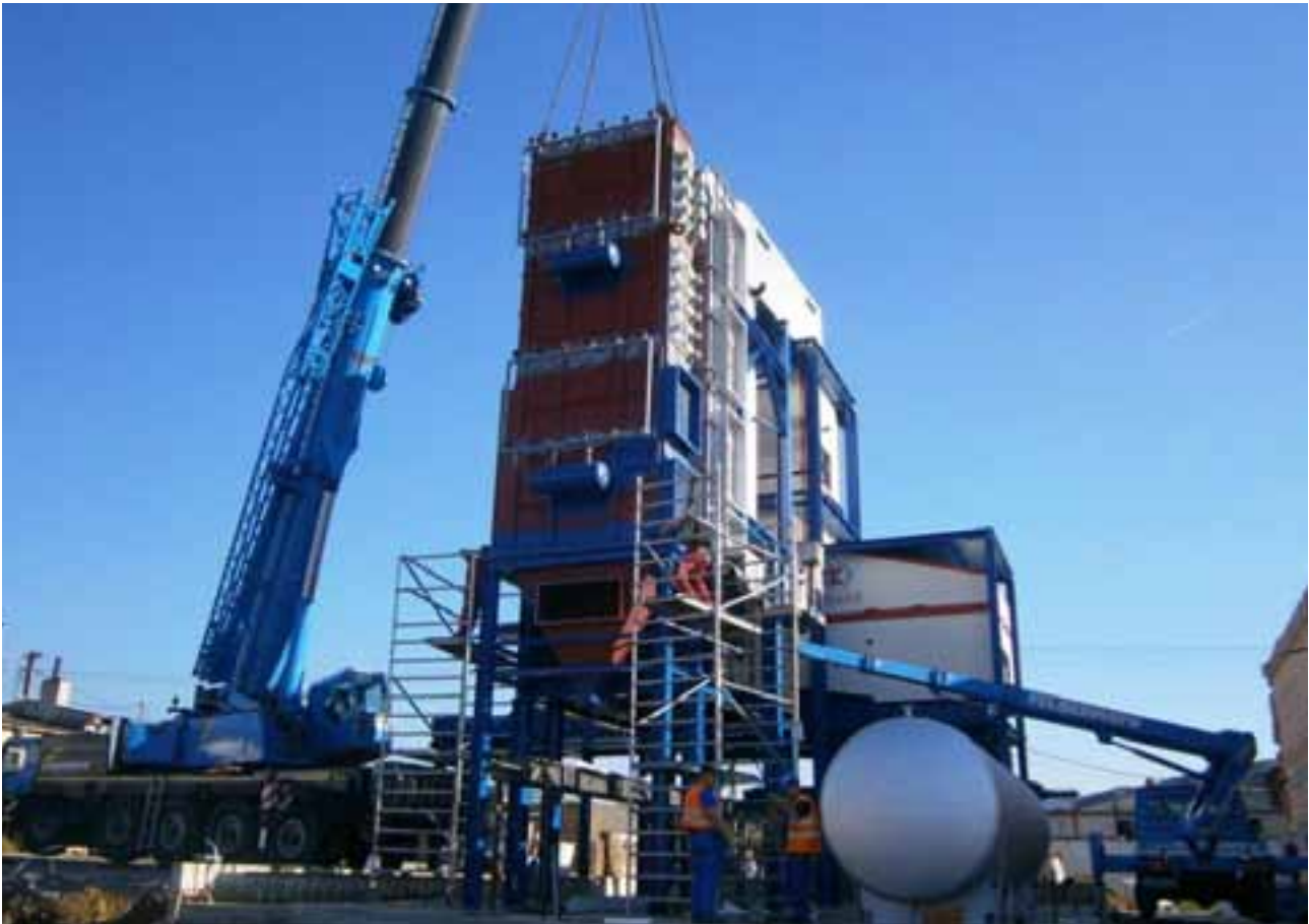
Figure 21 - Plant before realization
