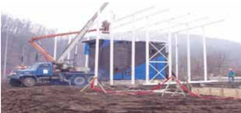
Figure 18 - Installation of biomass boiler
