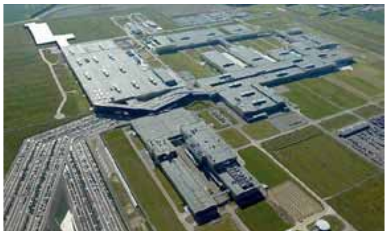
Figure 29: BMW factory in Munich
